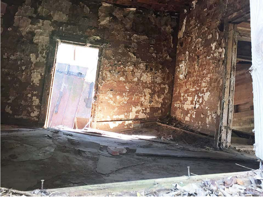
Fig. 3: Author photograph of an abandoned structure located behind campus. Alongside the anthropology department, students visit this location during a class meeting and take notes.
