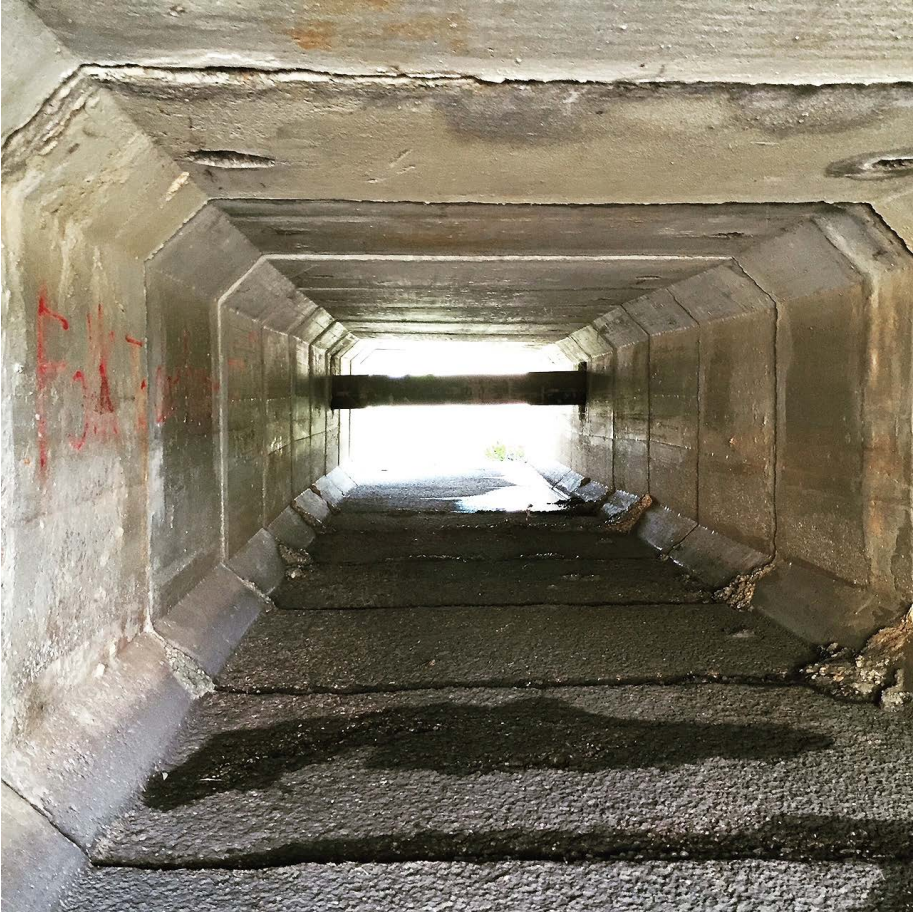
Fig. 4: Author photograph of a drainage tunnel beneath a neighborhood road.
