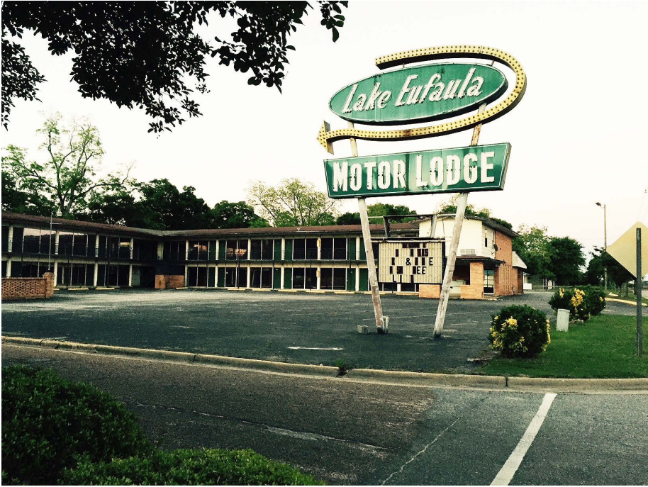
Fig 1: Author photograph of an abandoned motel in Eufaula, Alabama
